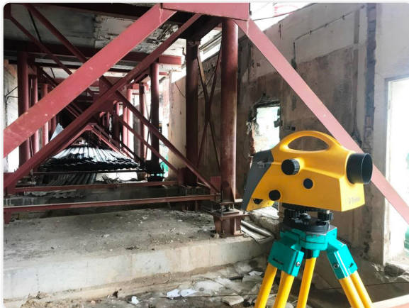
Fig. 18 Reinforcement of existing monolithic gallery structures
