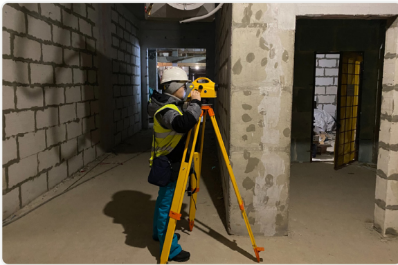
Fig. 14 Field measurements in the process of monitoring the precipitation of existing buildings and structures
