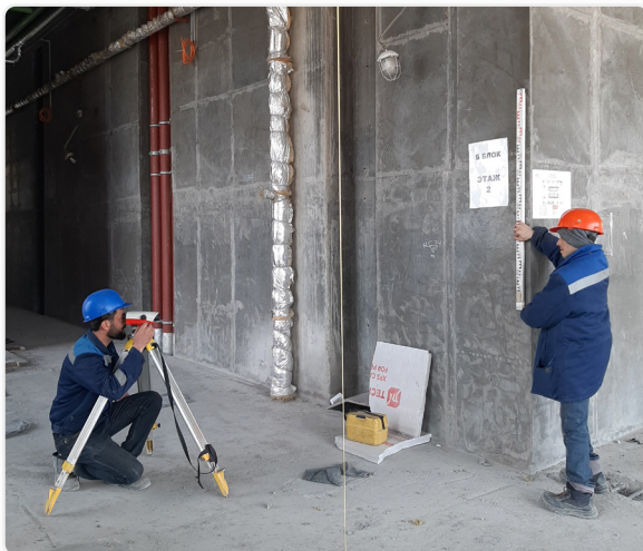
Fig. 26 The control of the removal of construction marks to the installation horizon
