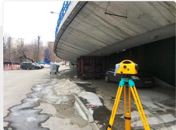
Fig. 19 Reinforcement of existing monolithic ramp structures
