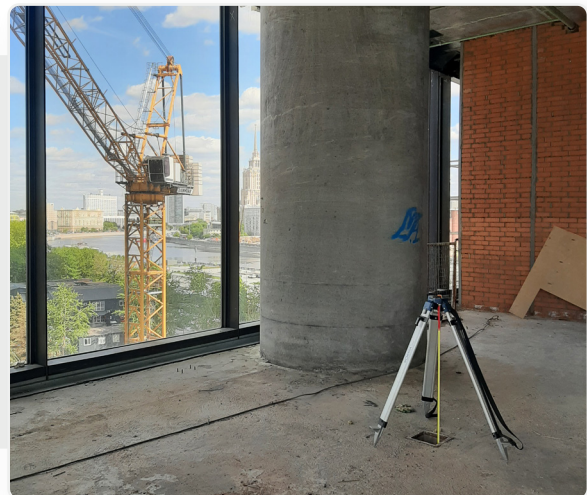
Fig. 26 The control of the removal of construction marks to the installation horizon
